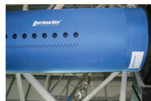
Round straight duct less than 9 m/s
