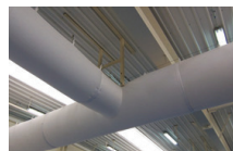
T connection less than 8 m/s
