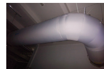
Elbow less than 8 m/s
