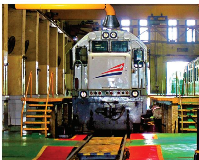
During maintenance and operating of diesel locomotives, they releases very hazardous gases. In order to this it should be efficiently absorbed and evacuated without spreading into the environment.
